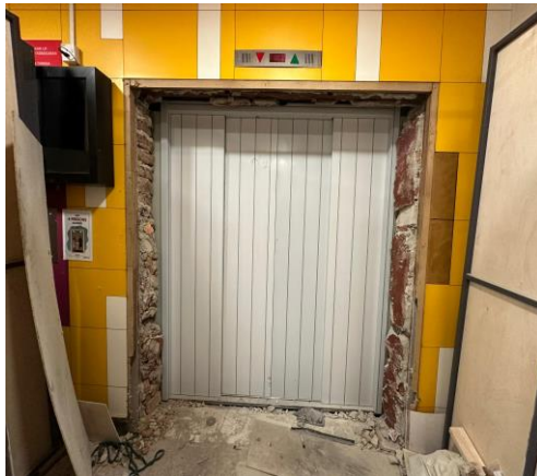
Installation of new lift landing doors, lift systems and structures
