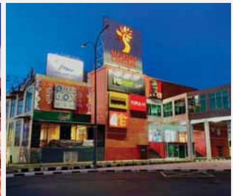
SEGAMAT CENTRAL Segamat, Johor Acquired in 2017 Valuation: RM65.0 million
