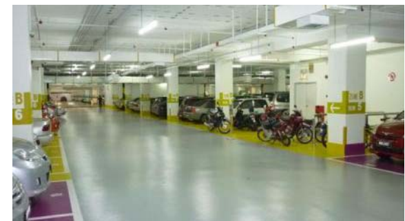
Basement Car Park
