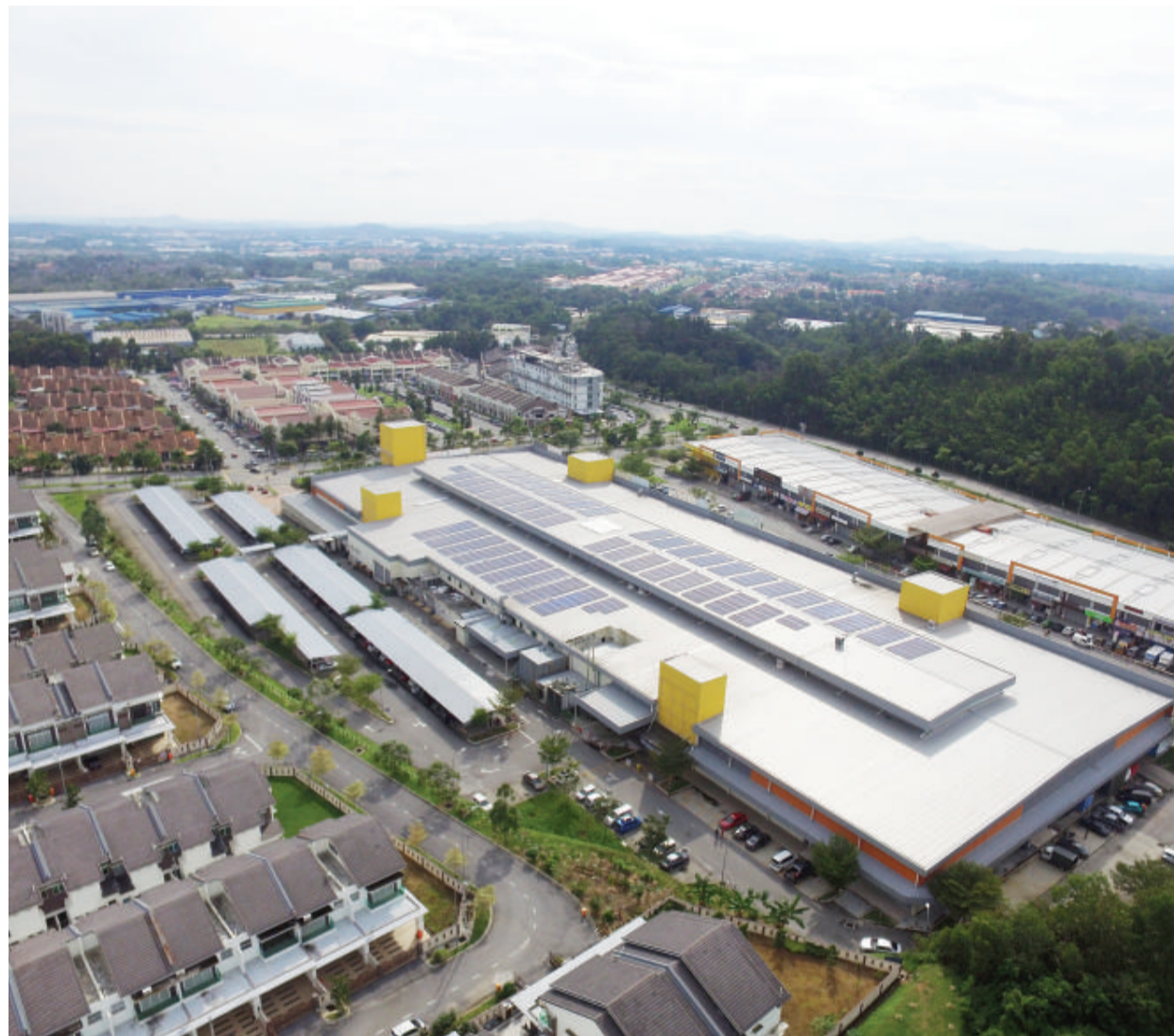
Solar PV system on KIP Mall Senawang. All KIP REIT's assets in the country had been fitted with a 2.73MWp solar PV system by last April
